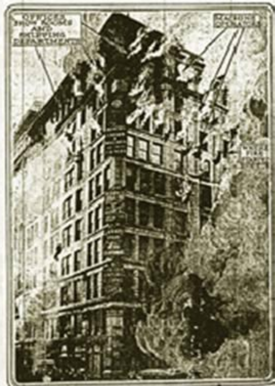
BUILDING AT NORTHWEST CORNER OF EAST WASHINGTON STREET AND GREENE STREET, FROM WHICH TOP FLOORS IN WHICH LOSS OF LIFE OCCURRED WERE COMPLETELY DESTROYED.
